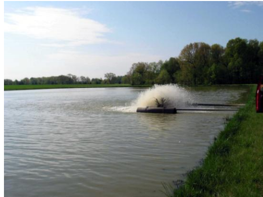
Steel paddlewheel aerator
