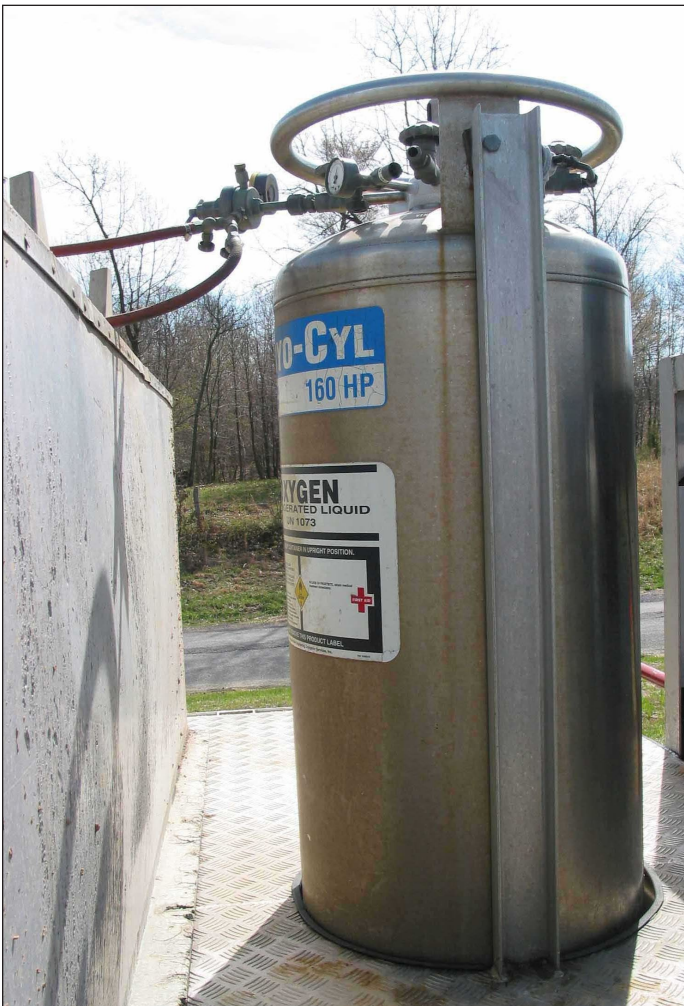
Figure 6. Liquid oxygen (LOX) dewar.
