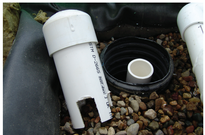
Figure 4. A bell siphon chamber (left) and stand pipe inside a permeable pipe (right).
